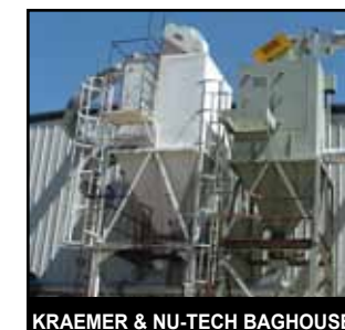
KRAEMER & NU-TECH BAGHOUSES
