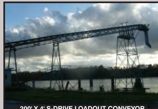
200' X 4' S-DRIVE LOADOUT CONVEYOR
